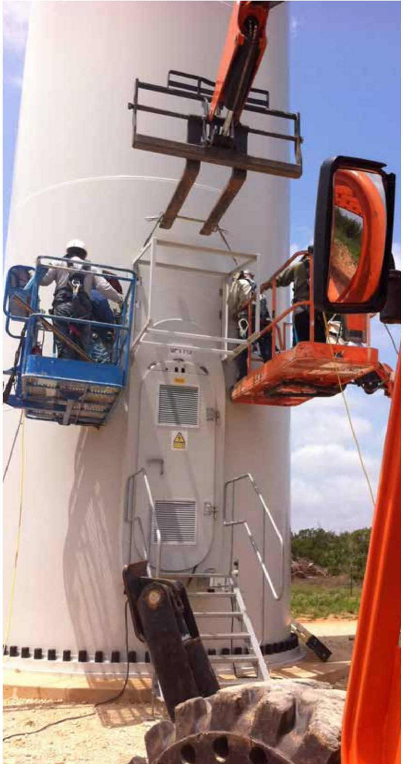
A weld team installs cooling system 100+ WTC.
