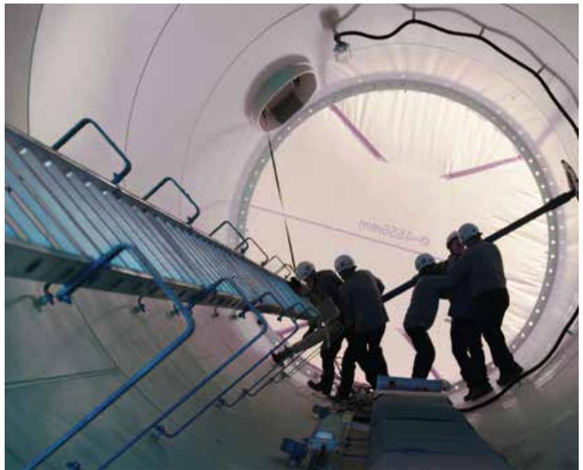
A dent crew sets up tooling in a section that was damaged. (Photos courtesy: BARR Fabrication Field Services)
